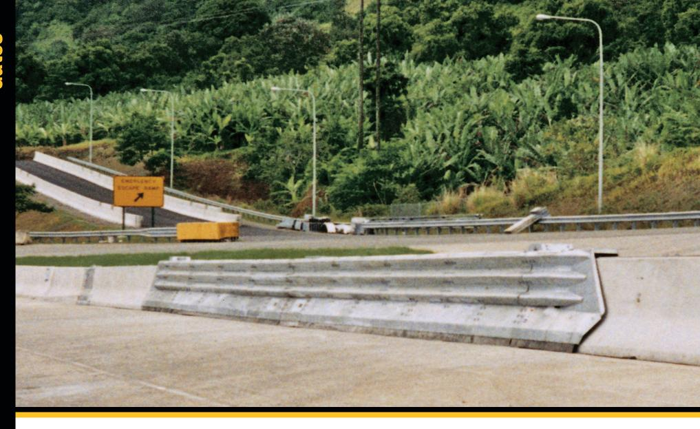
**BarrierGate**® Longitudinal Barrier Gate
